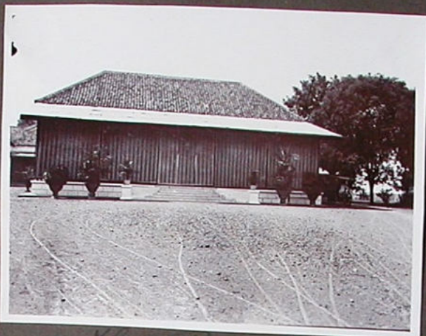
This Sarapattan 40 headquarters, constructed in 1926.
